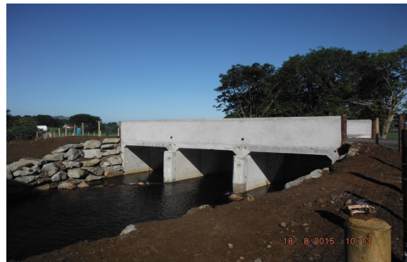
Straths Bridge, Inishowen – on completion
