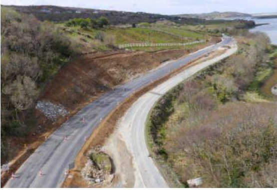
Realignment at the Gweebarra Bends on N56 in progress
