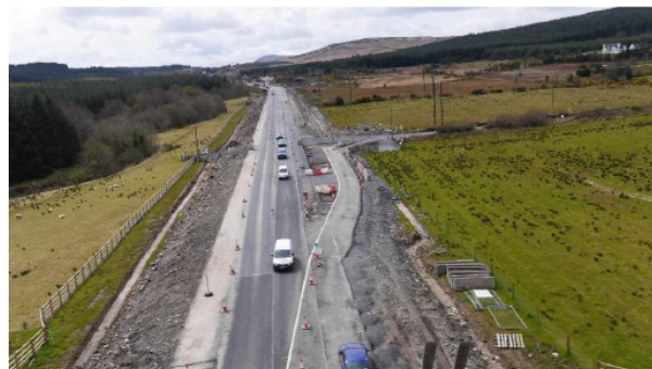
Blackburn Bridge Realignment Scheme – construction in progress
