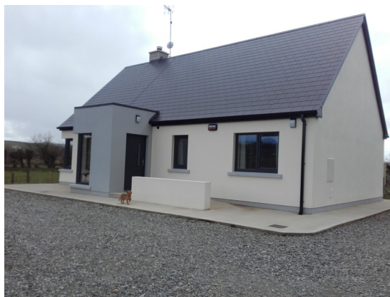
Specific Instance Rural Cottage at Monclink completed in 2015
